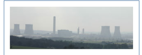
Didcot Power Station, August 2005.
